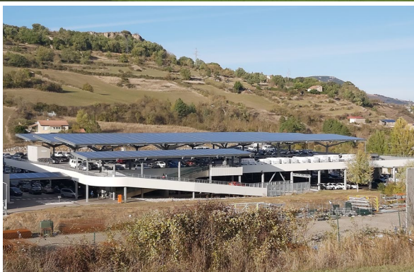
Ombrière de parking, Creissels (12). © Étienne Louyriac
